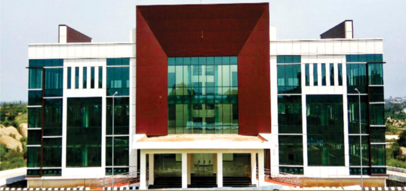
IT cum Administrative Building in operation, space available
