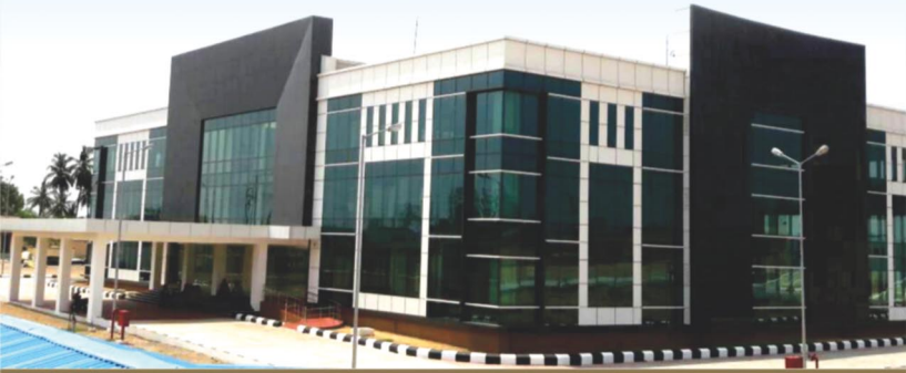
IT cum Administrative Building in operation, space available
